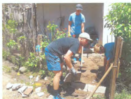
Our team helping build a new porch
